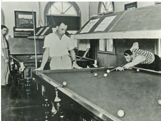
Police recreation room in the old Roma Street police station.
